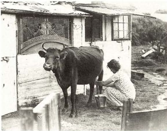
Top. Makeshift accommodation on permissive occupancy site at Happy Valley, near La Perouse, Sydney.
